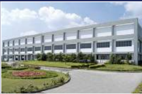
Aluminum Die Casting & Steel Fittings, Pune, India
