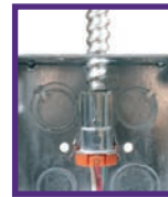
Step 2 Snap conduit into the fitting
