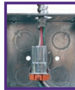
Step 1 Pull conduit thru knockout, insert wires into fitting
