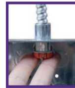
Step 3 Push fitting and conduit back thru knockout
