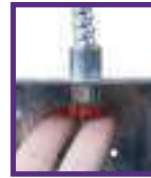
Step 3 Push fitting and conduit back through knockout
