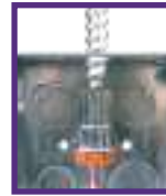
Step 2 Snap conduit into the fitting
