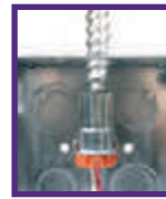
Step 2 Snap conduit into the fitting
