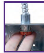
Step 3 Push fitting and conduit back thru knockout
