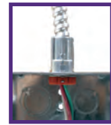
Step 4 Snap into knockout from inside the box
