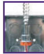
Step 2 Snap conduit into the fitting
